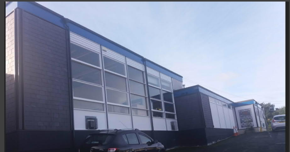
Single storey modular frame building
