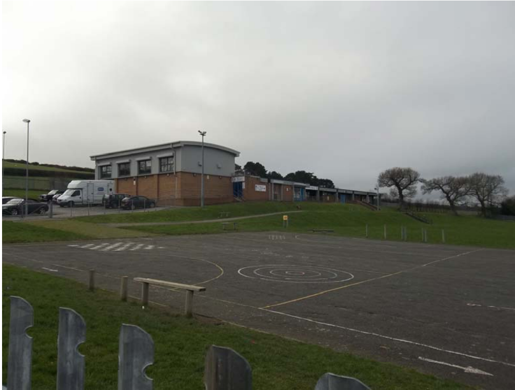
Figure 1 – Photograph of Existing School and Site
