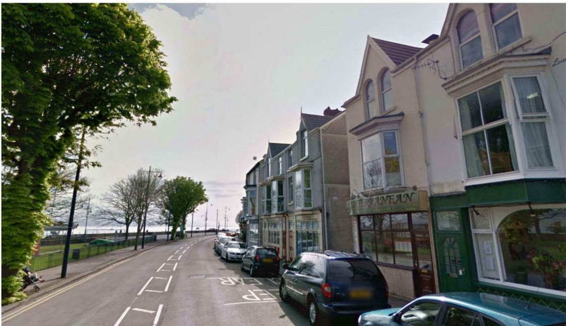
The inappropriate use and mixed styles of PVCu windows disrupts the street scene which give this terrace an uncared for appearance
