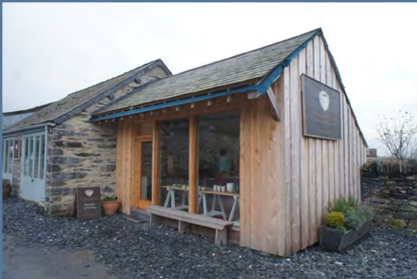
The Natural Building Centre, Llanrwst
