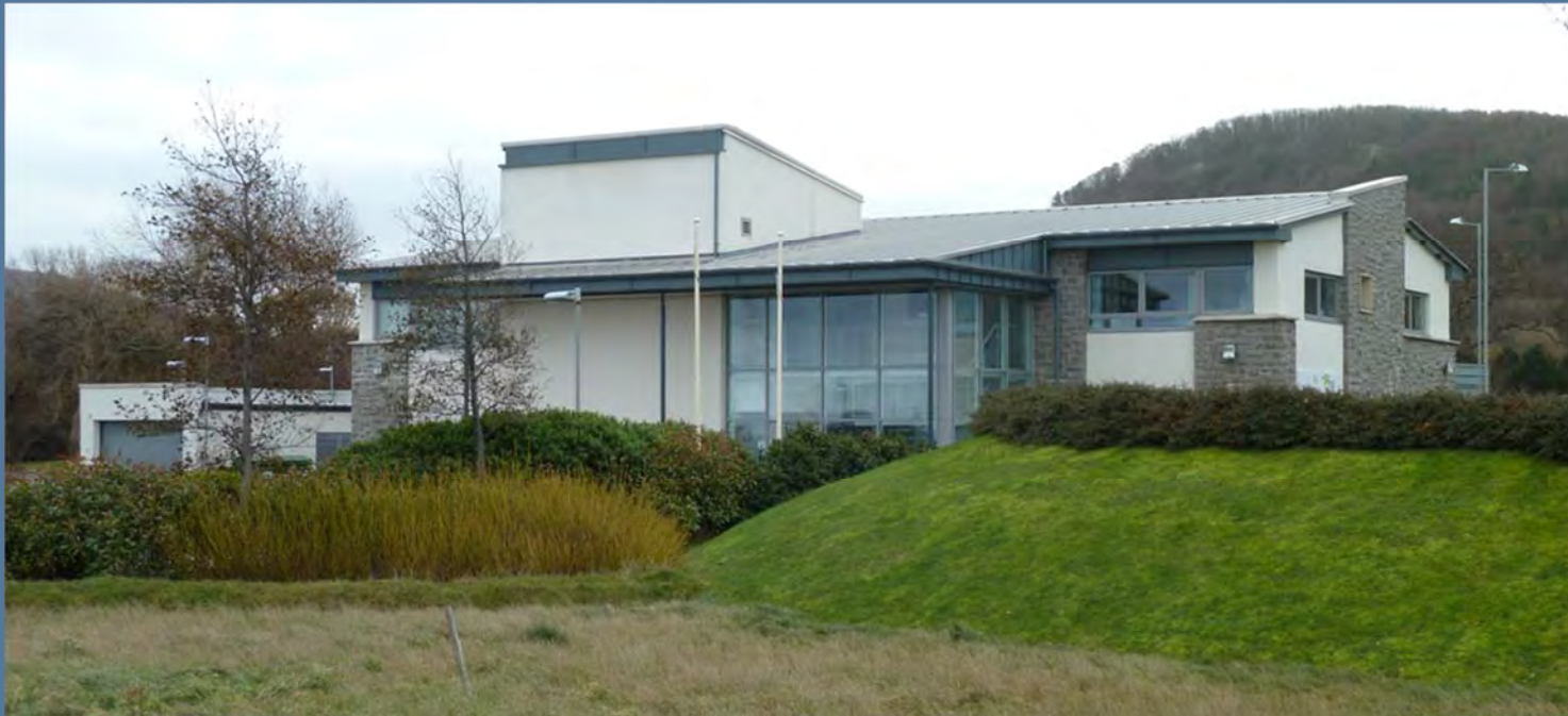
Abergele Business Park
