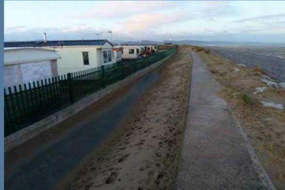
Image: Key issues in this photo are the high density of poorly sited static units. Note: no landscaping within site, screening or protection and also coastal processes underestimated and not accommodated for causing ongoing maintenance issues such as vandalism and damage to the statics and removal of sand from NCR5.
