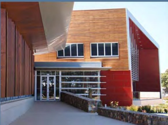
Image: Shire of Augusta office Margaret River , WA.
